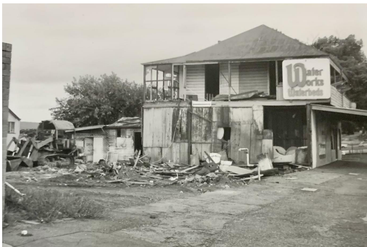
1988 Demolition of this row of shops underway
