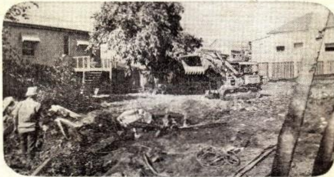
Bulldozers clear La Boite site. The tent is behind the tree.
