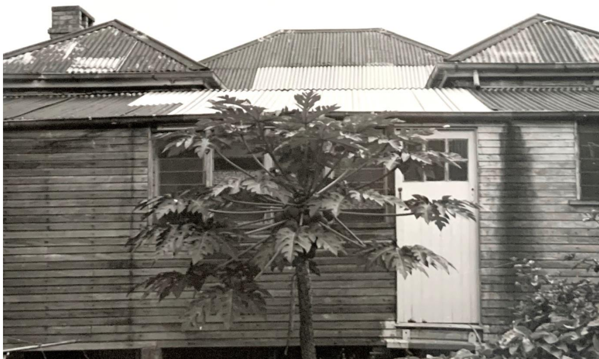
c1982 (Clyde Street 'frontage')
