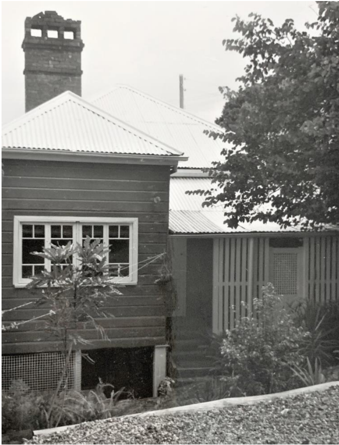
c1982 (Clyde Street 'frontage')
